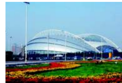
Shenyang Olympic Sports Center
