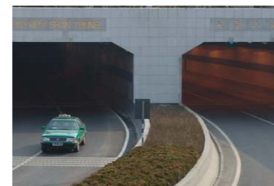
Nanjing Jiuhua Mountain Tunnel
